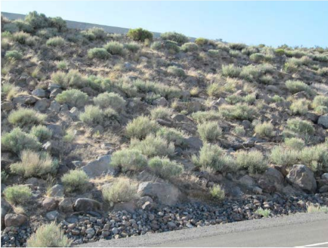
FIGURE 4 – REVEGETATED RIPRAP AREAS (TYPICAL)
