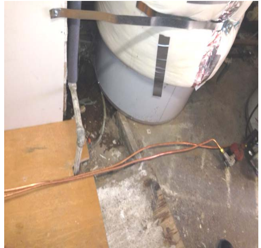
Kerosene fed into furnace 15' away
